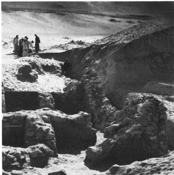
c) Wall slightly inclining inwards — (middle right)
