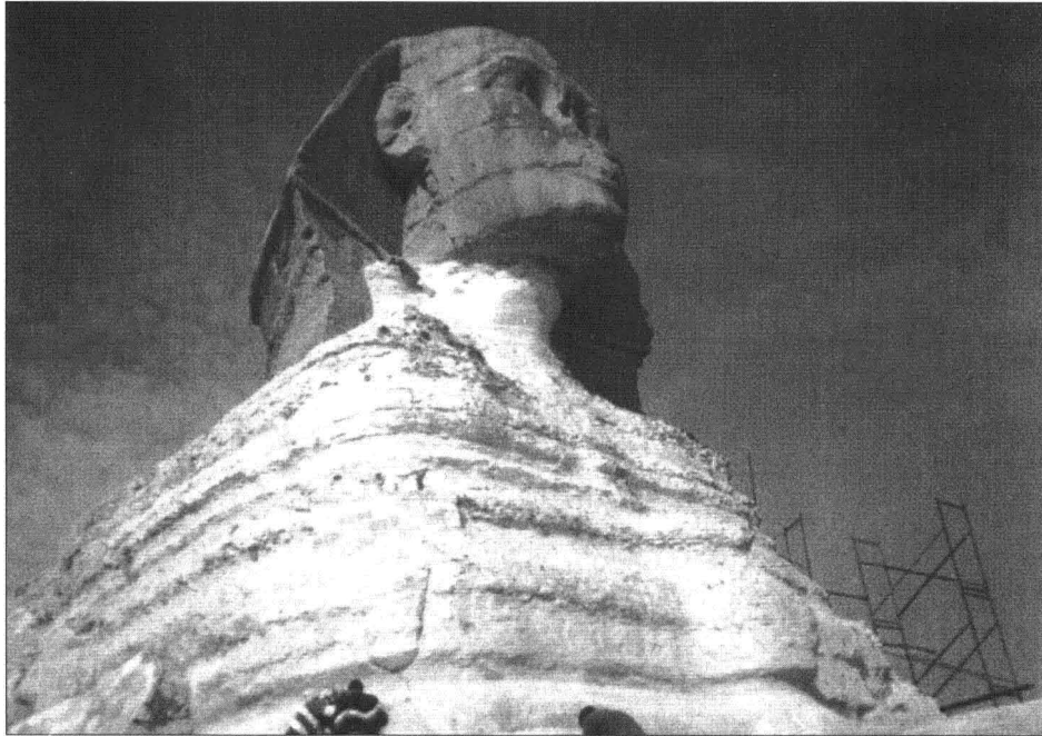
Fig. 3. View showing the weaker limestone in the neck.
